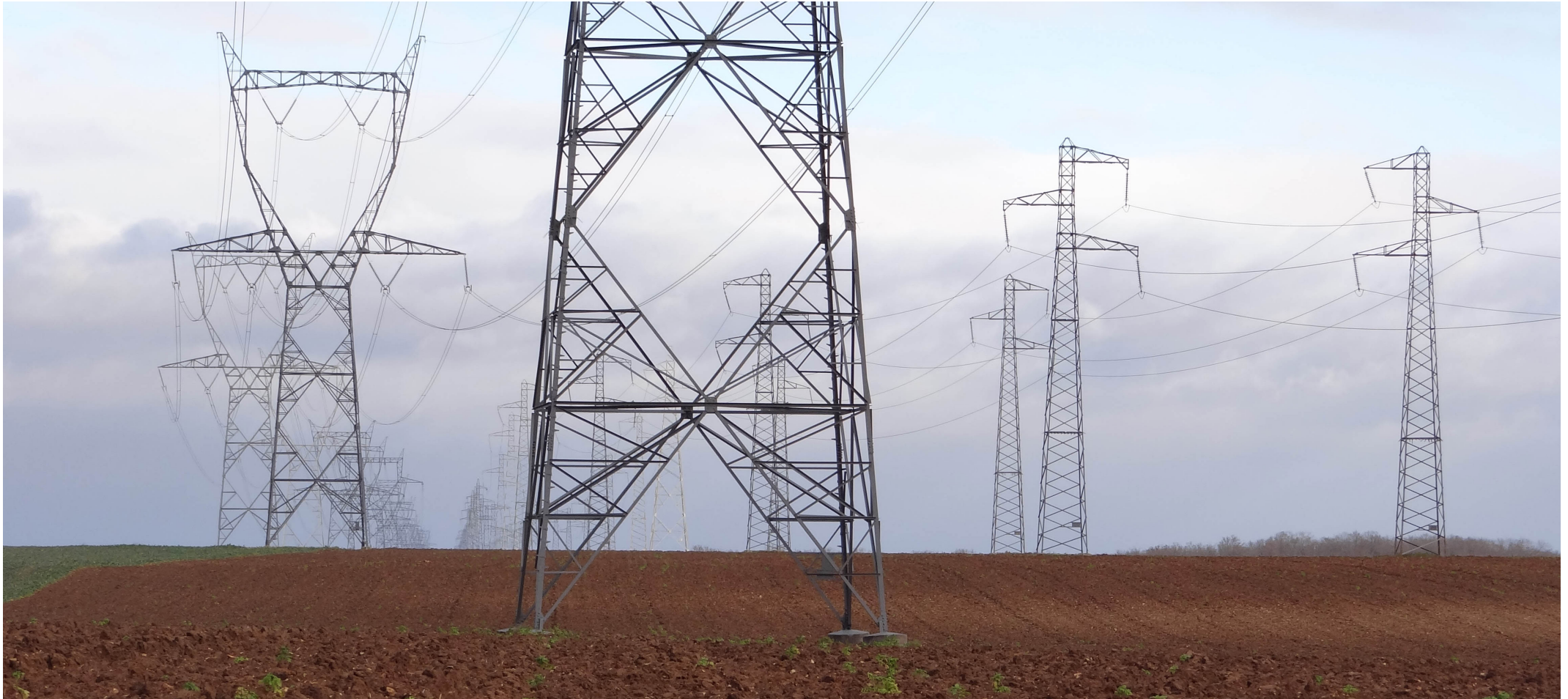
Chalou-Moulineux - Route de Thionville [Fig.1]
