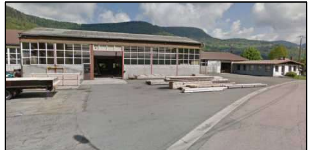
Hans coffrage, route de la Haitroye
