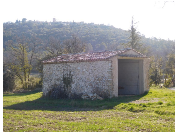
133. Hangar agricole, Ploungue, F 142
