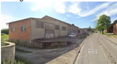
Ancienne station essence/garage
