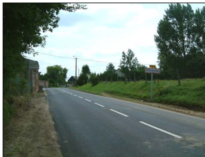
Photo 2. Entrée de village Sud, route D 23
