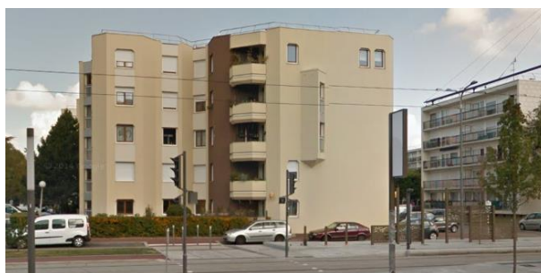
Logements SEMIV, avenue Louis Breguet
