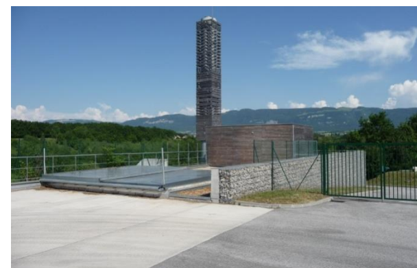
Chaufferie collective bois – Route des Primevères
