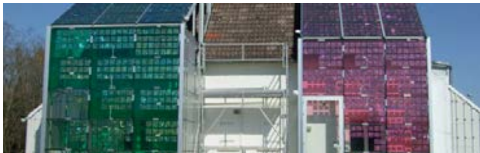
Prototype double peau photovoltaïque, ETI Construction, 2015
