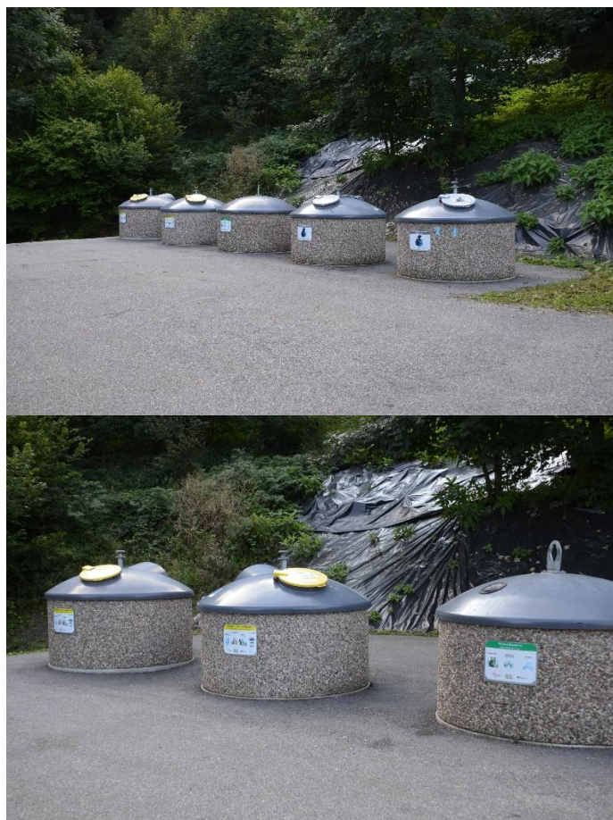
Conteneurs semi-enterrés de Montsapey (photo Luc Laurent)
