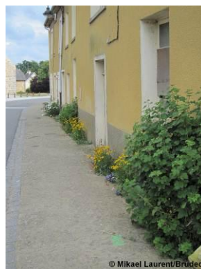
Trottoir accessible PMR – La Chapelle Thouarault (35) ▶
