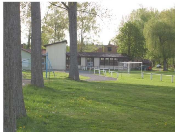
25.Club-house + terrain de football
