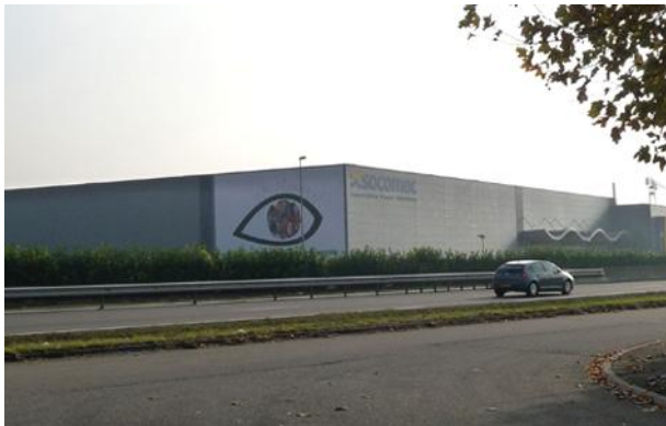
RD 1083 – Ets Socomec
