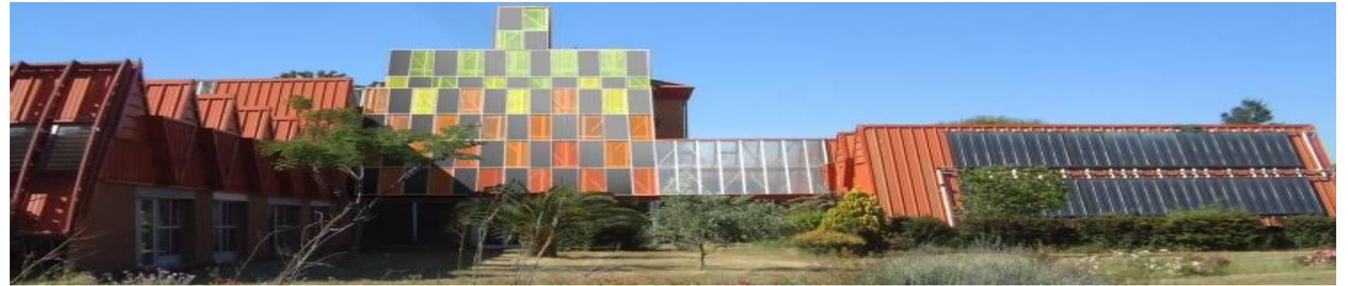
Photo 35: Lycée agricole Federico Garcia Lorca
