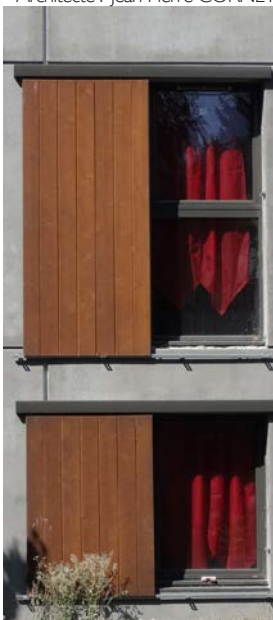
Panneaux bois coulissants (Magny-en-Vexin)
