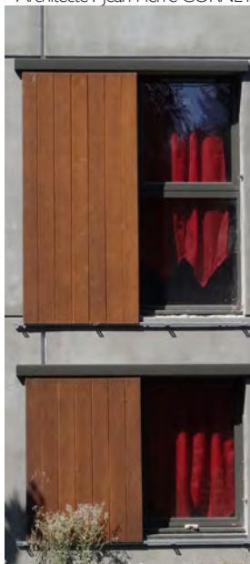
Panneaux bois coulissants (Magny-en-Vexin)
