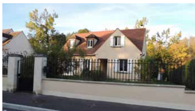
Pavillon - Source: Cabinet Gossart
