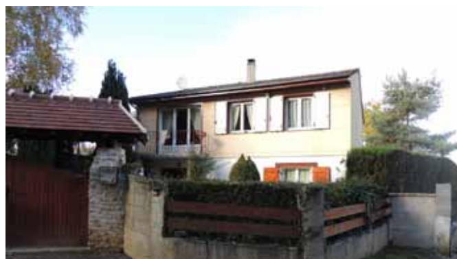
Pavillon - Source: Cabinet Gossart
