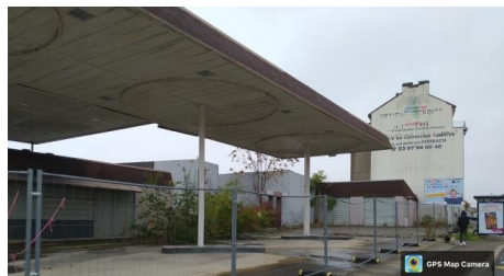
Ancienne station service avenue Saint-Rémy
