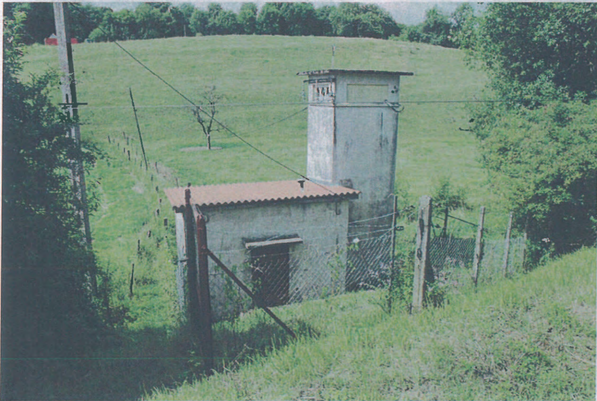
Le captage - la station
