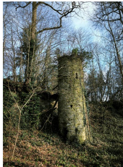
Station de pompage
