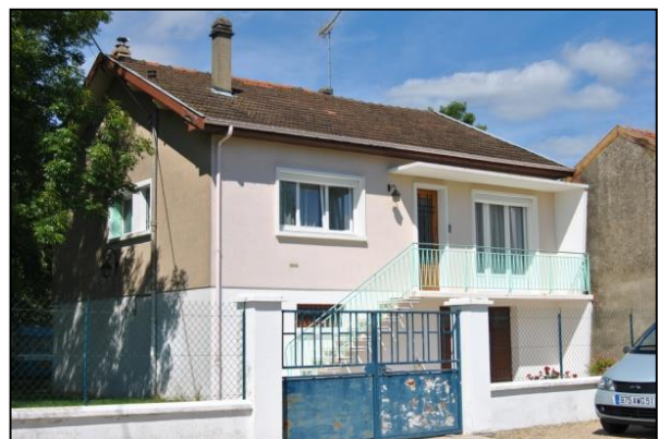
Pavillons Source TOPOS
