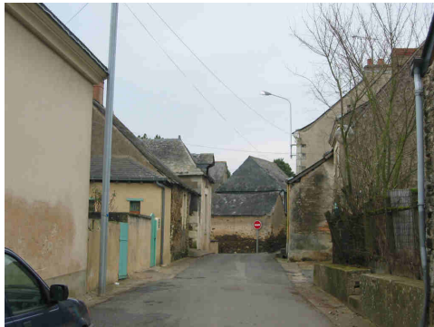
Imbrication des constructions
