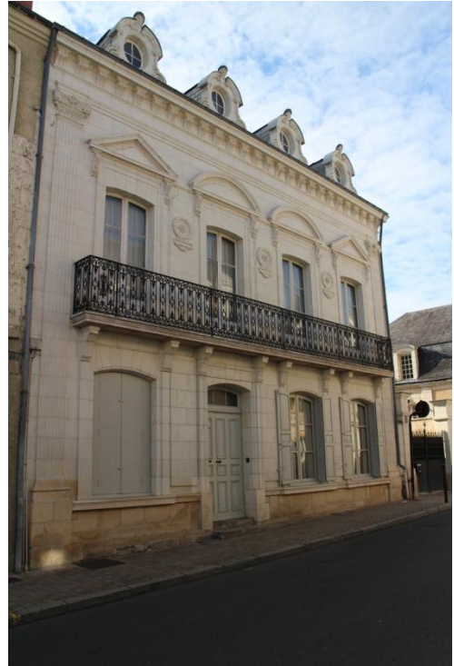
Balcon filant, Baugé
