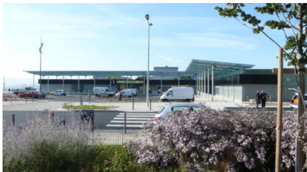
Centre commercial Vivaldi
