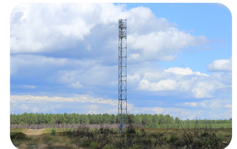
Antenne-relais Source : ARTIFEX 2023
