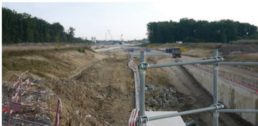
La construction de la LGV (Ecopertica, 2013)
