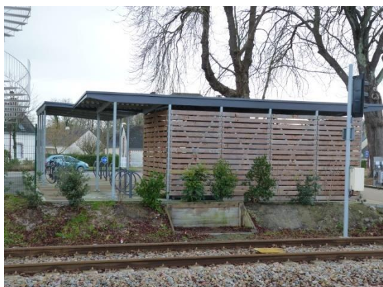
Parking vélo – Gare multimodale – Sucé-sur-Erdre (44)
