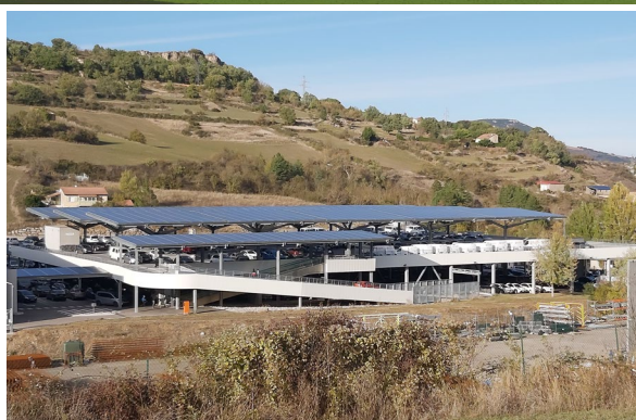
Ombrière de parking, Creissels (12). © Étienne Louyriac
