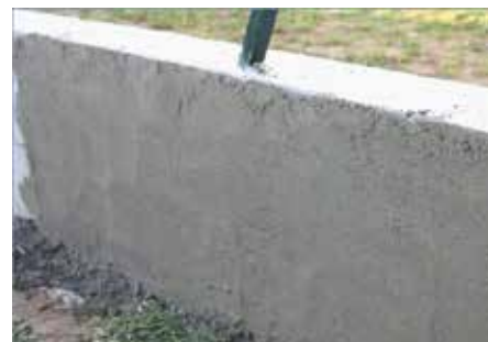
Mur parpaing - habillage ciment
