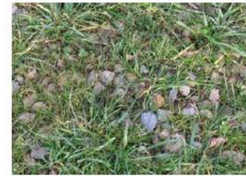
parking terre-pierre enherbé
