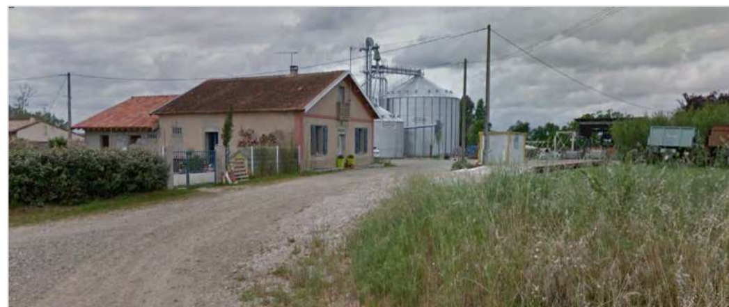
Figure 32 : silos route de Launac, source Google
