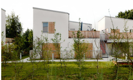
Dumont Legrand Architectes, Saint-Jean-de-Braye (45) - RDC+1
