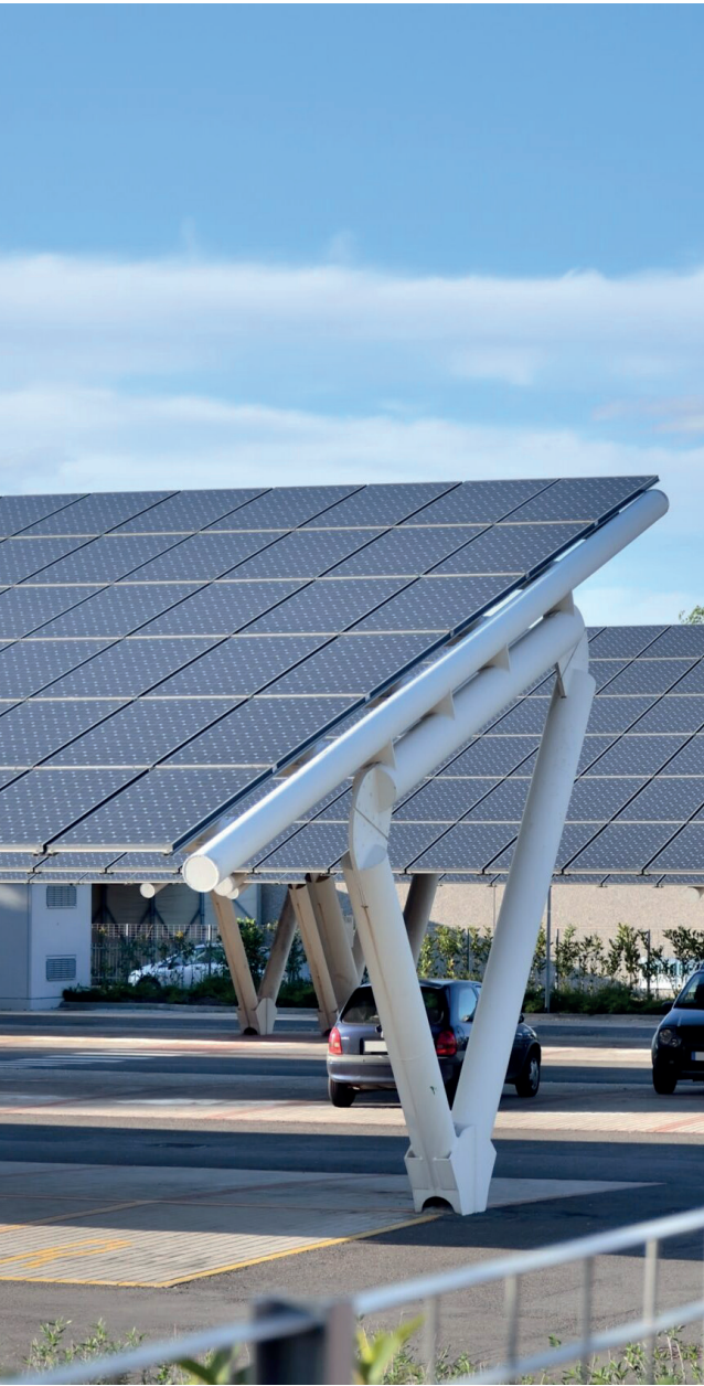
Parking couvert d'ombrières photovoltaïques
