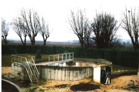
Figure 56 La station d'épuration intercommunale
