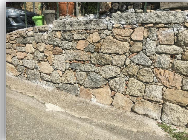
Image 4 (muret 2, Village d'Arbellara 07/2018)
