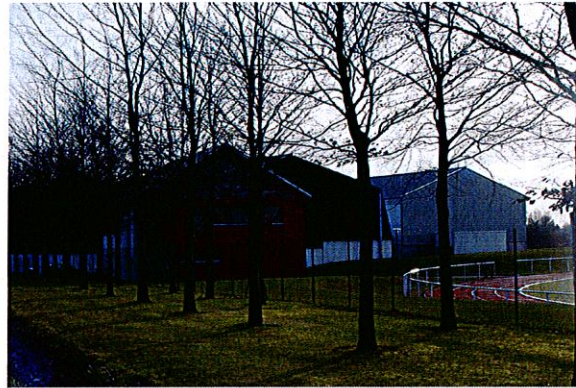
Figure 5: Caserne de pompiers
