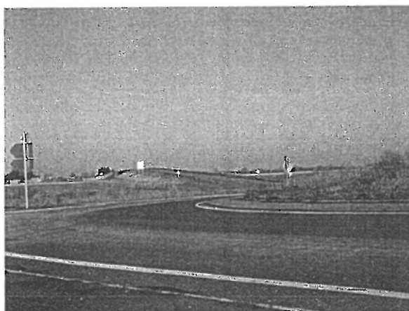
Figure 15ter: Infrastructures de la RD 438
