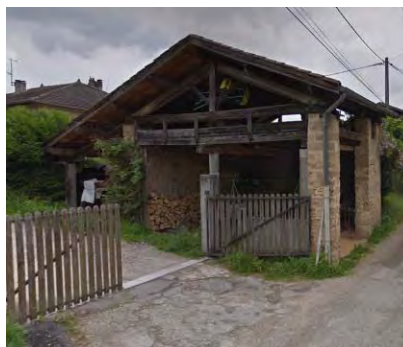
24 – Architecture agricole, les Macaires Remise agricole
