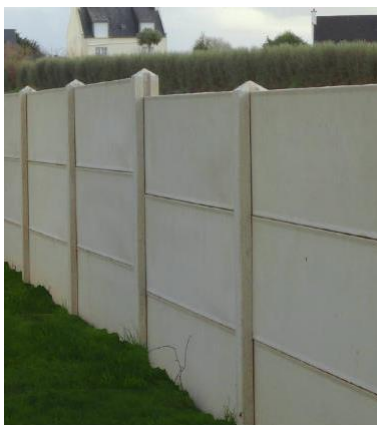
PLAQUES LISSES BETON MOULE
