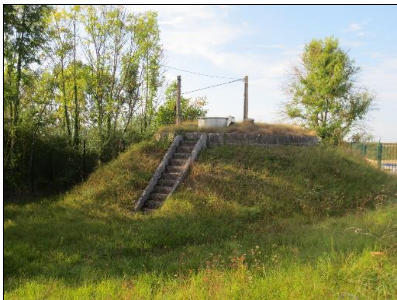
13. Cuve semi-enterrée (80 m 3 )
