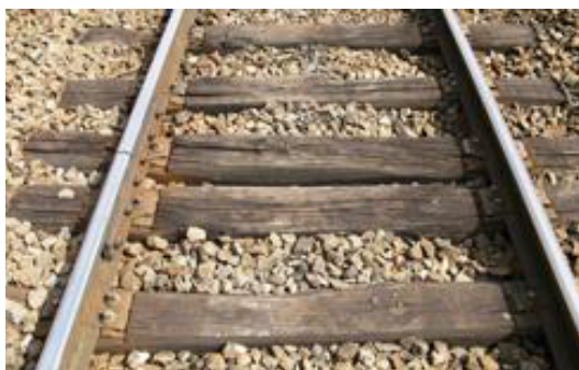
Figure 36: Rails courts sur traverses bois
