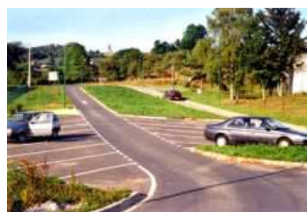
Zone de parking existante
