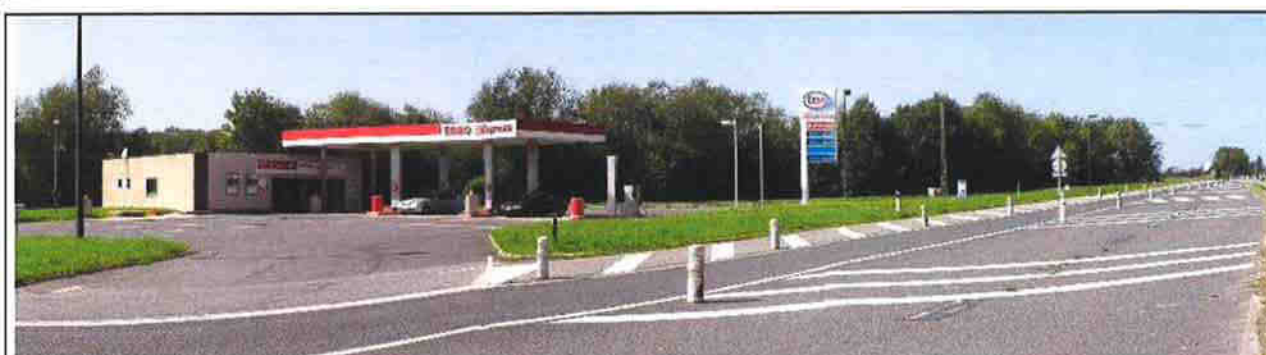
La station de distribution de carburants
