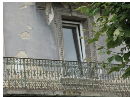
Garde corps balcon
