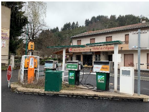
Station essence, source : IATE
