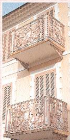
Façade de village
