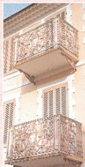
Façade de village
