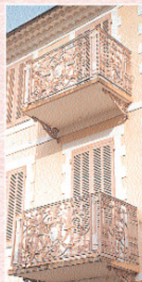
Façade de village
