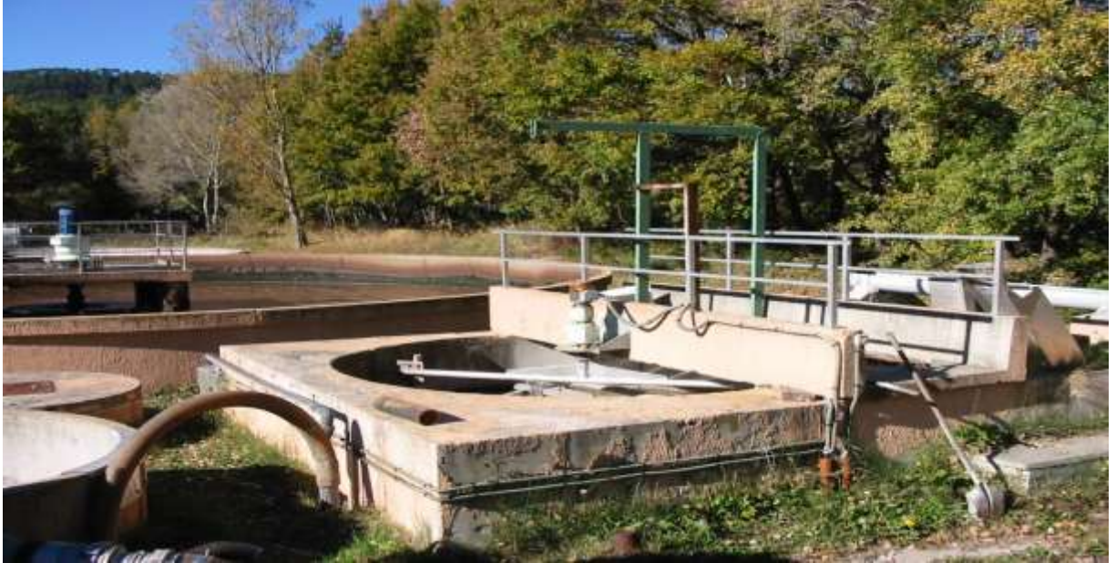
Figure 2-1 : Station d'épuration de Moustier Sainte-Marie
