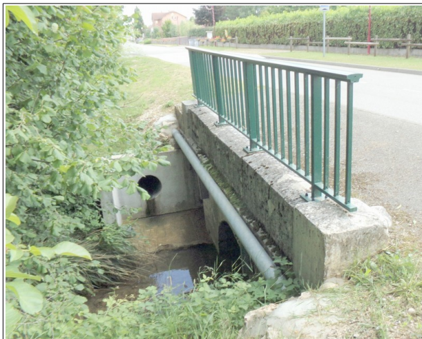
Figure III.63: pont de la RD984
